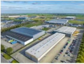
Steel structure warehouse
