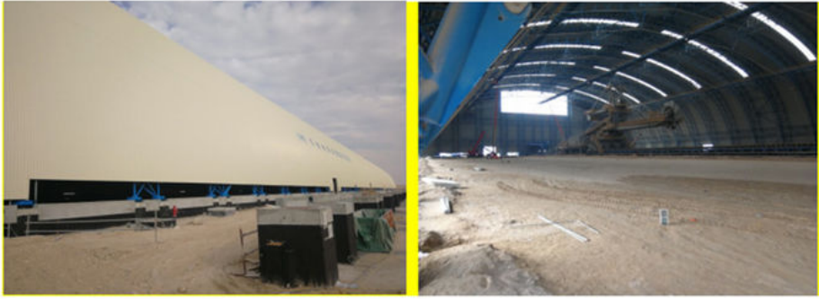
Clean Coal Fired Power Plant Phase I (4x600mw net) Project in Hasyan Dubai
