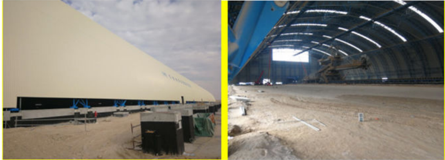
Clean Coal Fired Power Plant Phase I (4x600mw net) Project in Hasyan Dubai
