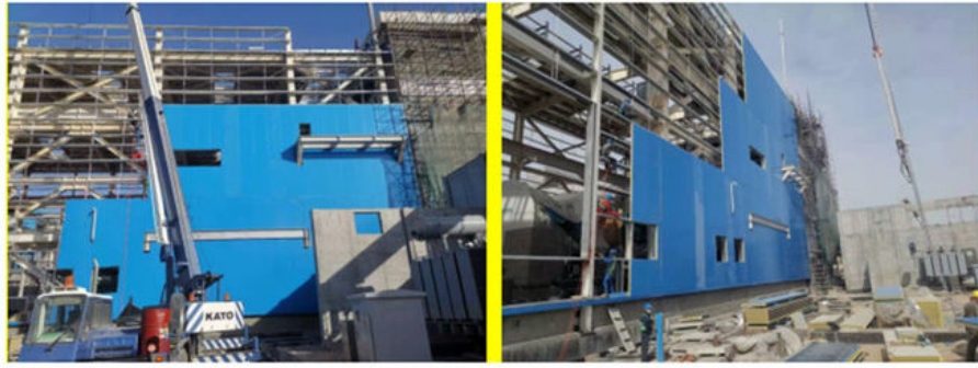
Gas Turbine Combined Cycle Power Station Expansion Project in Basra Iraq
